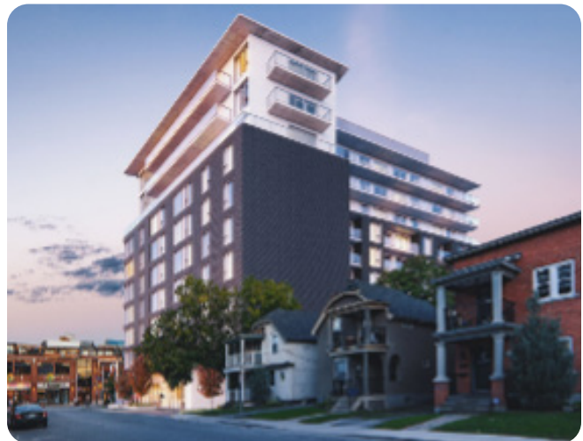
46 Flora Street, Ottawa A 114-unit purpose-built rental apartment built by Taggart, with majority of units meeting CMHC affordability criteria
