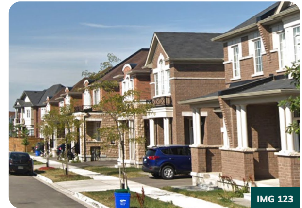
Set back garage doors from the entrances of low-rise dwellings to minimize their visual impact on the street.
