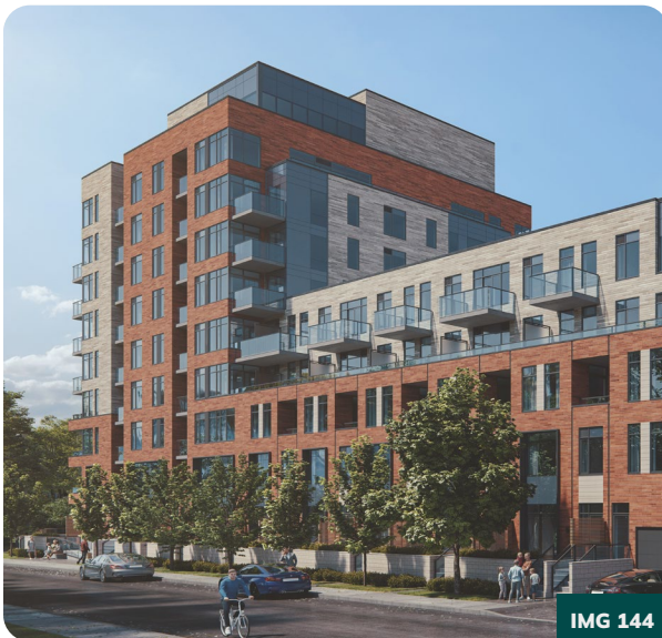
Taggart's development 93 Norman Street, Ottawa delivered a 122-unit purpose-built rental apartment offering affordable and large (2+ bedroom) units.
