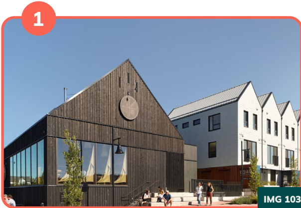
1 Buildings, regardless of typology or land use, should have a direct relationship with the community spine to create an active, vibrant corridor.
