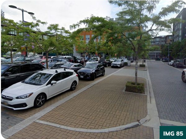
Where they exist, larger surface parking lots will be landscaped, include defined pedestrian connections and organized to support intensification over time.
