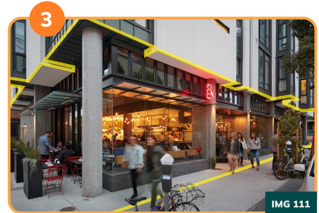
A variety of commercial formats will be permitted along the Community Spine, including mixed-use buildings with retail at grade and standalone retail. These uses should maintain an active frontage along the Spine and key pedestrian routes.
